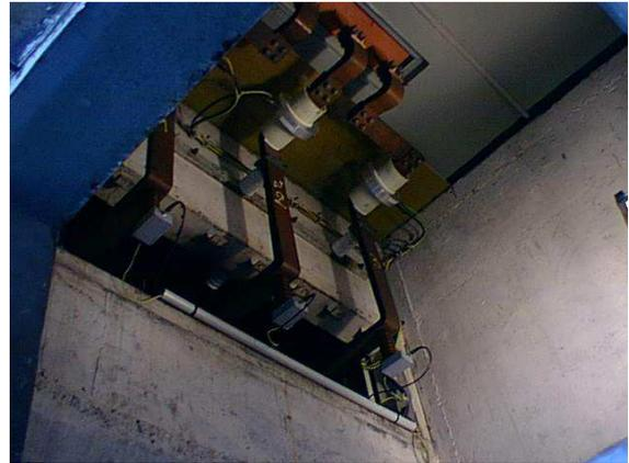
Picture: 16 MW synchronous motor connections hall, ROGOWSKI coils at the top and divise capacitors at the bottom
