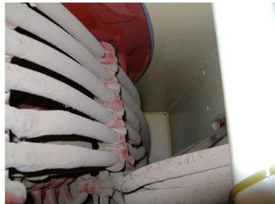
Fig. PD activity on HV induction motor (Air Liquide)
